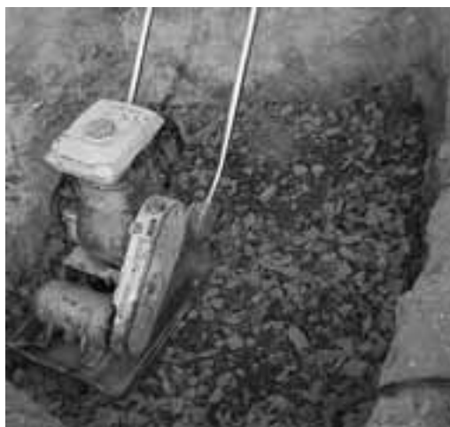
Figure 1 Test pit (gravel)
