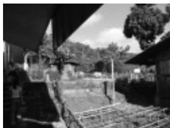
View of the compound from the staff house
